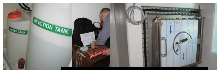
Chemical Effluent Decontamination Systems must be validated by the user (left), pressure charting: No excursions into positive pressure are allowed according to BMBL 2007 for BSL-3 facilities (middle), BSL-3 autoclaves must have true bioseals (right).
