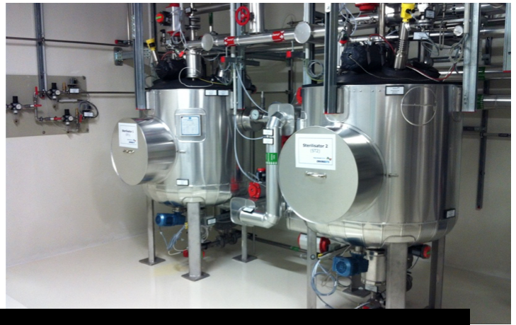
Left: HEPA-filtration housing. Right: Redundant thermal effluent decontamination system
