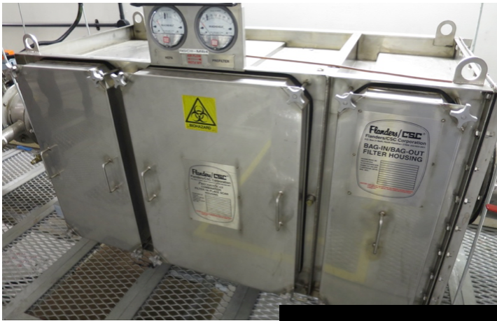
Left: HEPA-filtration housing. Right: Redundant thermal effluent decontamination system
